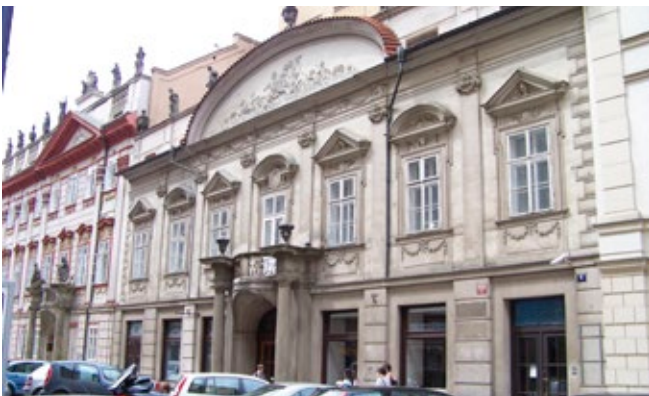
Historical building, offices Prague CZ, 2015 - CoolGRID
