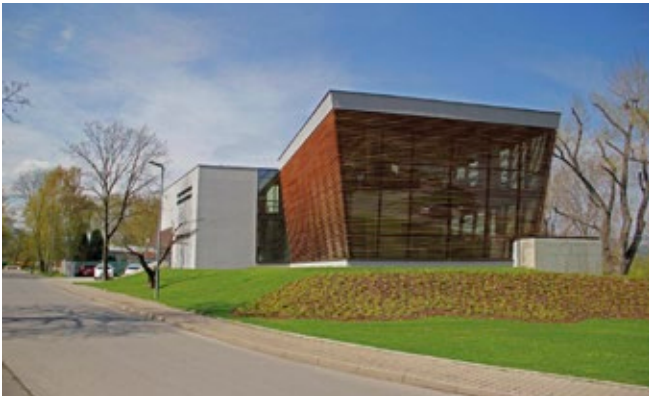
Training center Lovosice CZ, 2016 - CoolPLATE, CoolGRID
