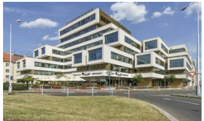
Office building QUBIX Prague CZ, 2010 - CoolGRID
